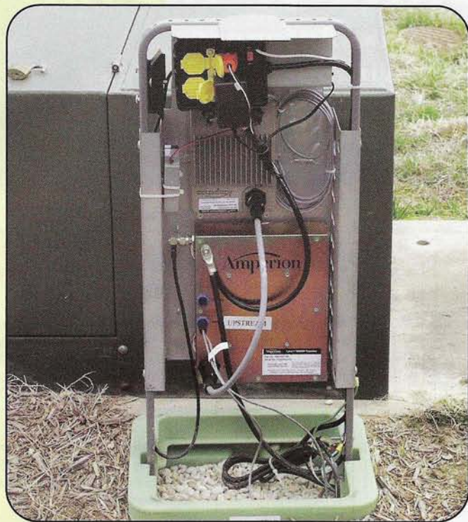
This is the BPL hardware inside the ground-mounted pedestal.
